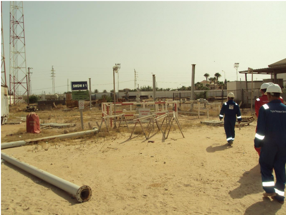
Figure All.17: Water Disposal Well SWDW#1
