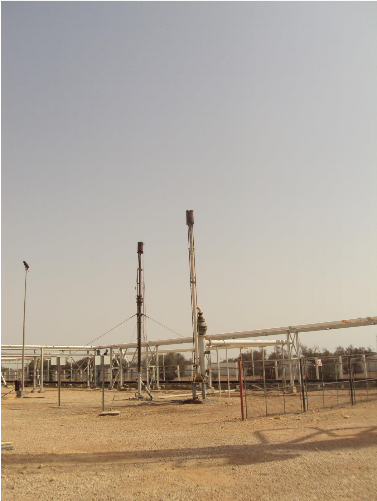
Figure All.6: Flares at Tank Battery
