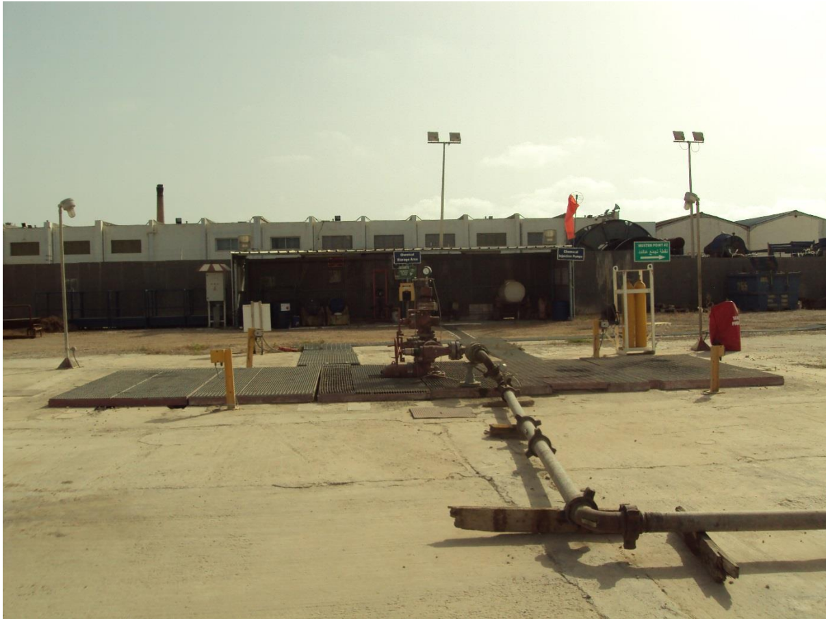
Figure All.13: Rhem01 Well Site
